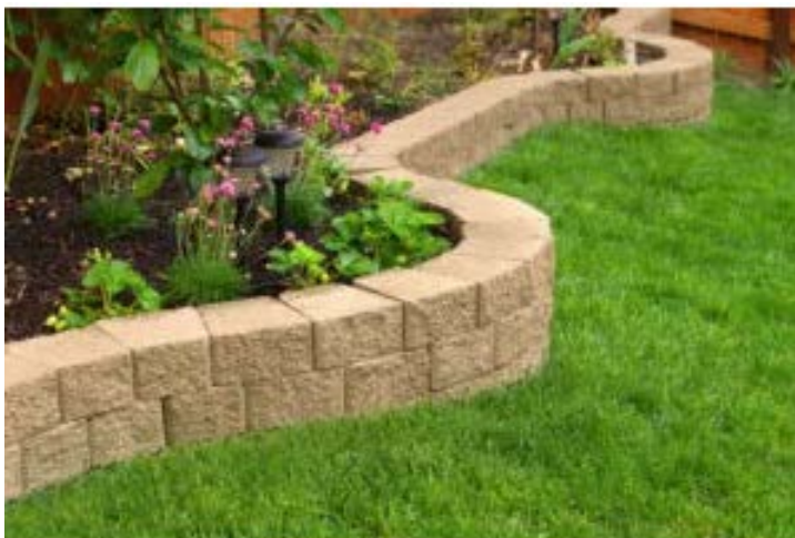
Figure 6 An example using landscape bricks
