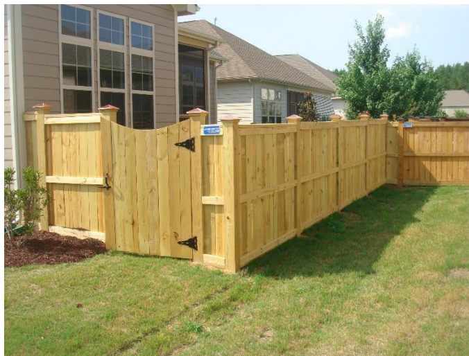
Figure 2 Approved Wooden Privacy Fence Installed by Harrison Fence
